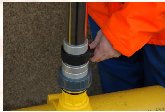
Push the dome downwards and secure the down by means of the lever.
