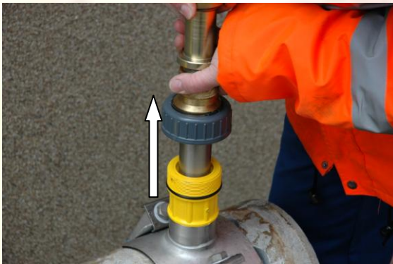
Remove the entire hot tap tool from the yellow POLSAFE valve.
