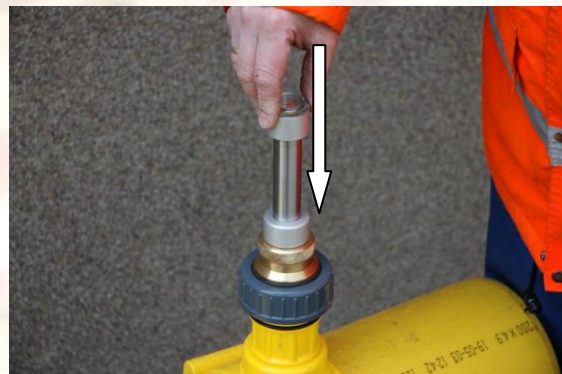
Push the flow direction meter completely downwards.
