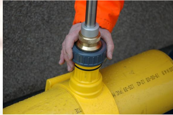
Install the flow direction meter into the yellow POLSAFE valve and secure the meter by turning down the bushing completely.
