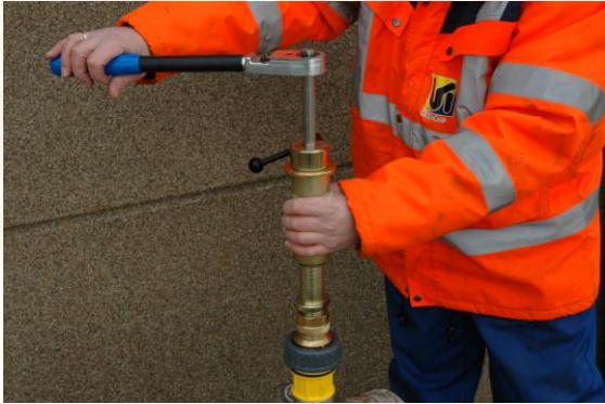
Start hot tapping the pipeline.
