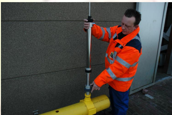
Install the dome onto the yellow valve.
